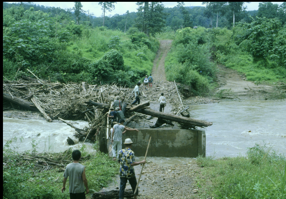
The bridge over the Nam Lang after a flood washed away the approach, the day before Mindy' seizure in 1991 (Close to the Edge).
