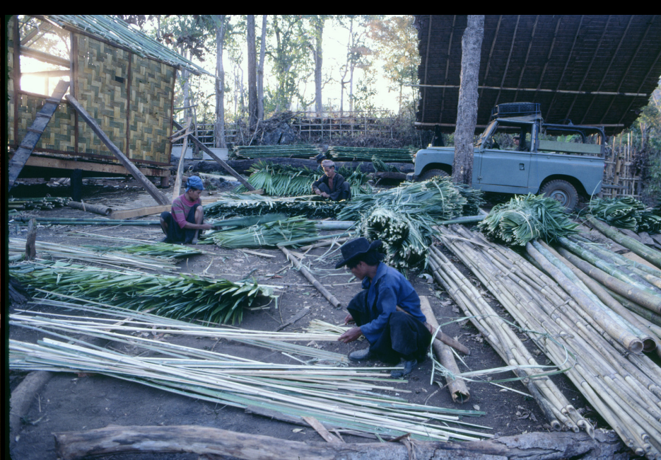
Black Lahu friends from Ban Huai Hea constructed our first roof in 1984 from bamboo and cabbage palm leaves (Head for the Hills).
